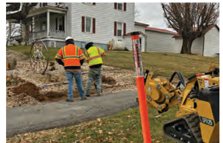
Crews install fiber in Middlebrook, Va.
