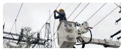
Of course, no one would ever purposely cause the death of a lineworker. Nevertheless, a generator connected to a home's wiring or plugged into a regular household outlet can cause backfeeding along power lines and electrocute anyone who comes in contact with them — even if the line seems de-energized.
